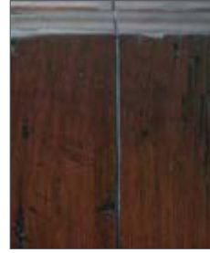
MEDIUM DISTRESS Shown on Plank Top
