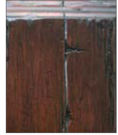
HEAVY DISTRESS Shown on Plank Top
