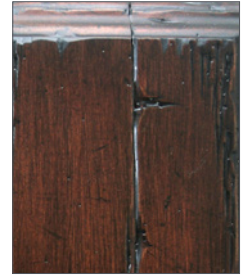
HEAVY DISTRESS Shown on Plank Top
