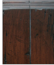
MEDIUM DISTRESS Shown on Plank Top
